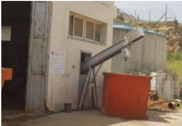
Figure 2: Al-Bireh WWTP, (a) shows dewatered sludge output and (b) shows aeration tanks
