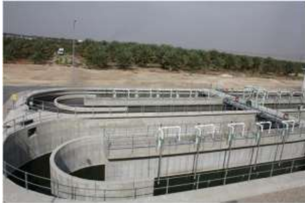
Figure 3 : Jericho WWTP, (a) shows aeration tanks and (b) shows sludge beds
