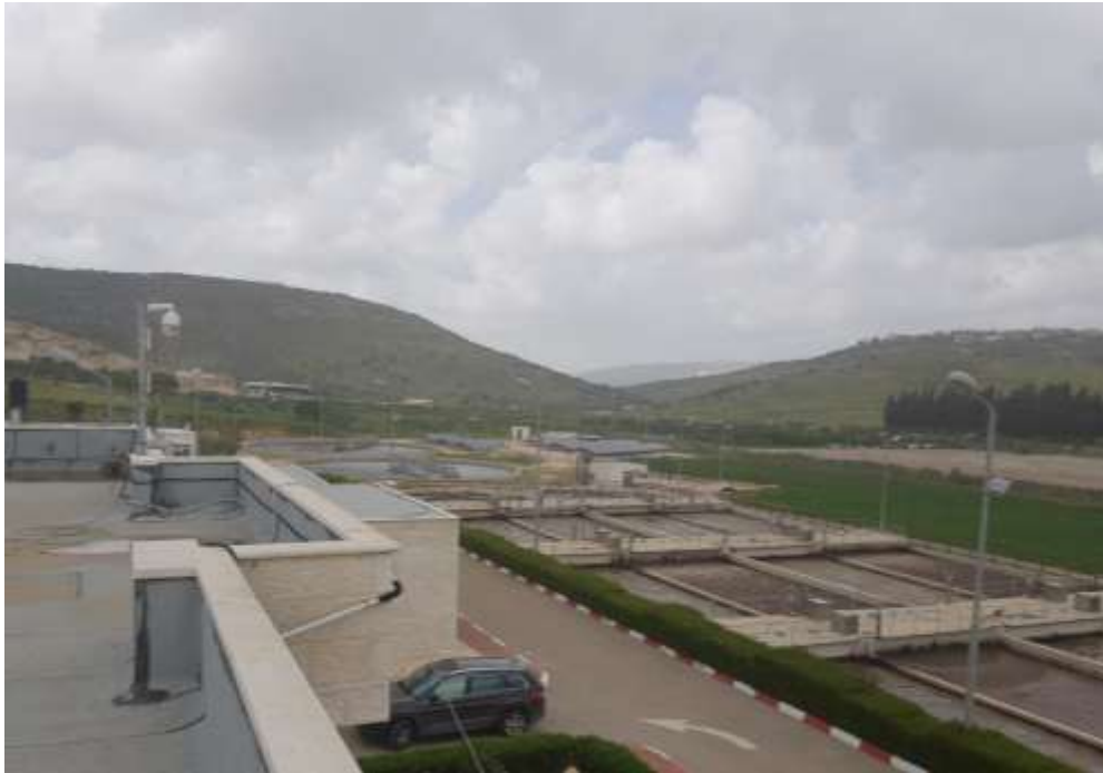
Figure 5: Nablus West WWTP (overview of the aeration tanks)
