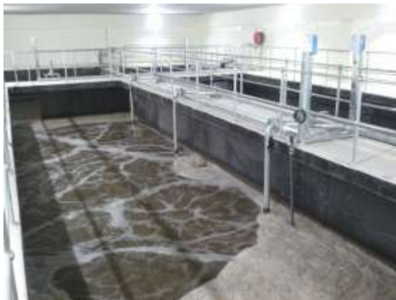
Figure 4: Al-Tireh WWTP, (a) shows aeration tanks and (b) shows the outside WWTP building.
